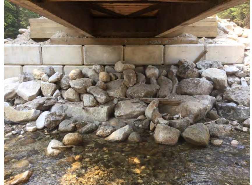
Right Bank Abutment when facing downstream
