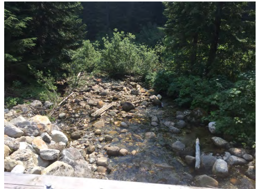
Looking downstream from deck
