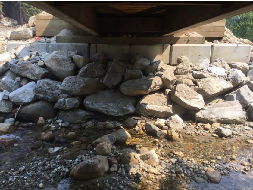
Left Bank Abutment when facing downstream
